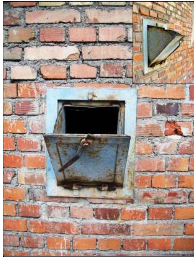
One of the two iron hoppers added later into the outside wall of the Dachau room claimed to have been a homicidal gas chamber.
